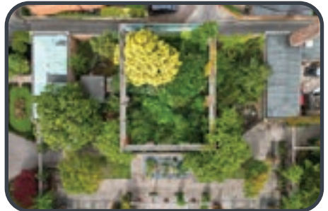
Aerial view of the Queen's Park Hothouse
