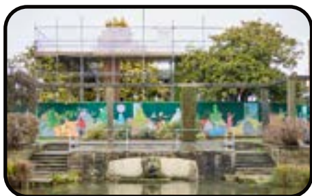
Hothouse remodelling work
