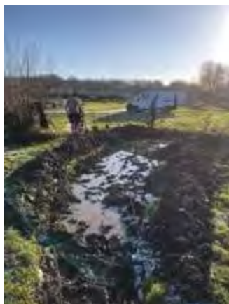
Construction of the new wildlife pond
